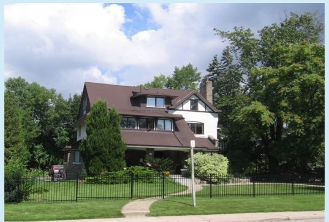
Figure B135 — 84 High Street East, CG Hamilton House, Designated
