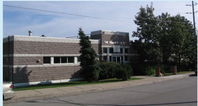
Figure B24 — Image of the Riverside Precinct
