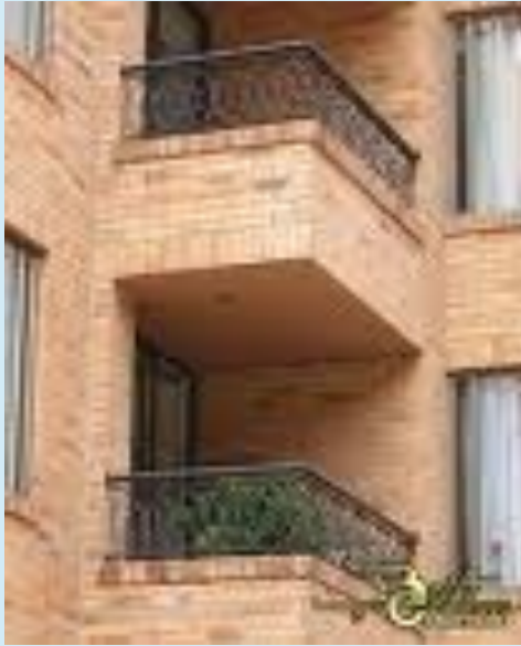
Figure 101 — Balconies should be designed so that they are part of the building rather than added onto the building as an afterthought. Glass balconies should have 50% tinting to ensure items on the balcony are not fully exposed
