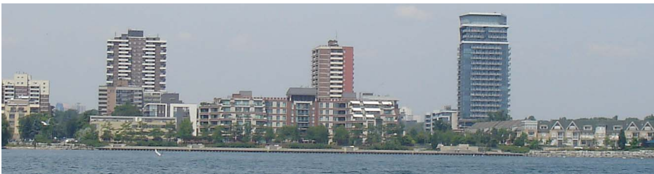
Figure 2: The Port Credit Node contains a range of building types, including: townhouses, mid-rise, and high rise buildings. The built form of the node generally transitions downwards toward the waterfront and stable residential neighbourhoods to the east and west. A limited number of high rise towers punctuate the skyline.
