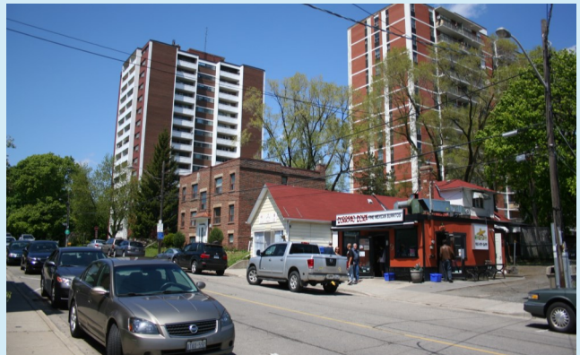
Figure B5 — Central Residential Precinct Image
