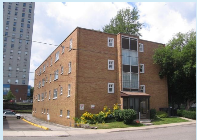
Figure B26 — Image of the Riverside Precinct
