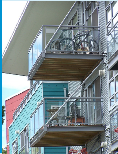
Figure 101 — Balconies should be designed so that they are part of the building rather than added onto the building as an afterthought. Glass balconies should have 50% tinting to ensure items on the balcony are not fully exposed
