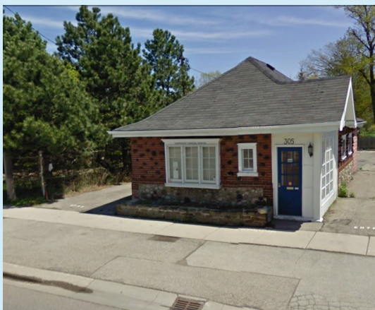
Figure C48 — 305 Lakeshore Road West Designated
