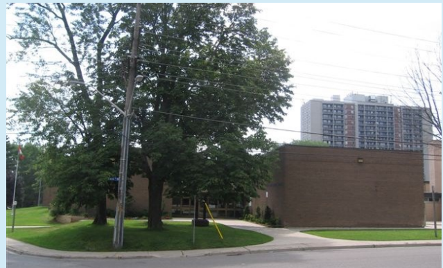
Figure B74 — Image of the Riverside Precinct
