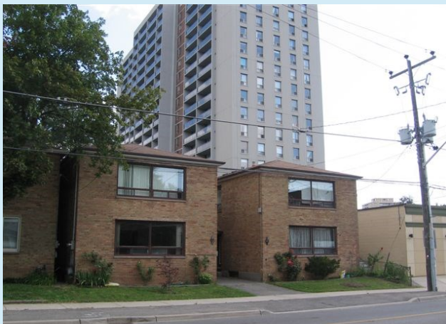
Figure B25 — Image of the Riverside Precinct
