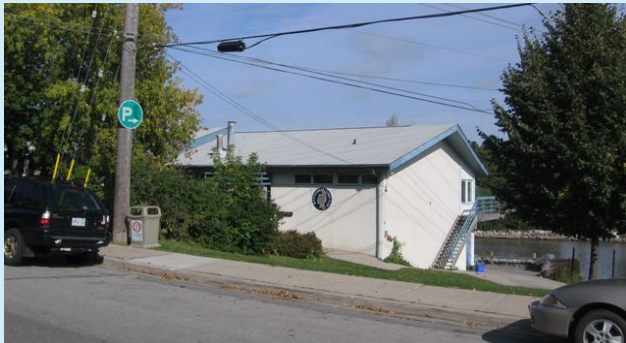
Figure B23 — Image of the Riverside Precinct
